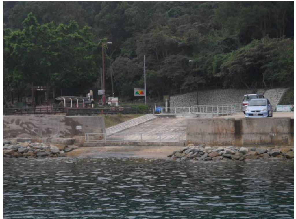
Example: Wong Shek Slipway
