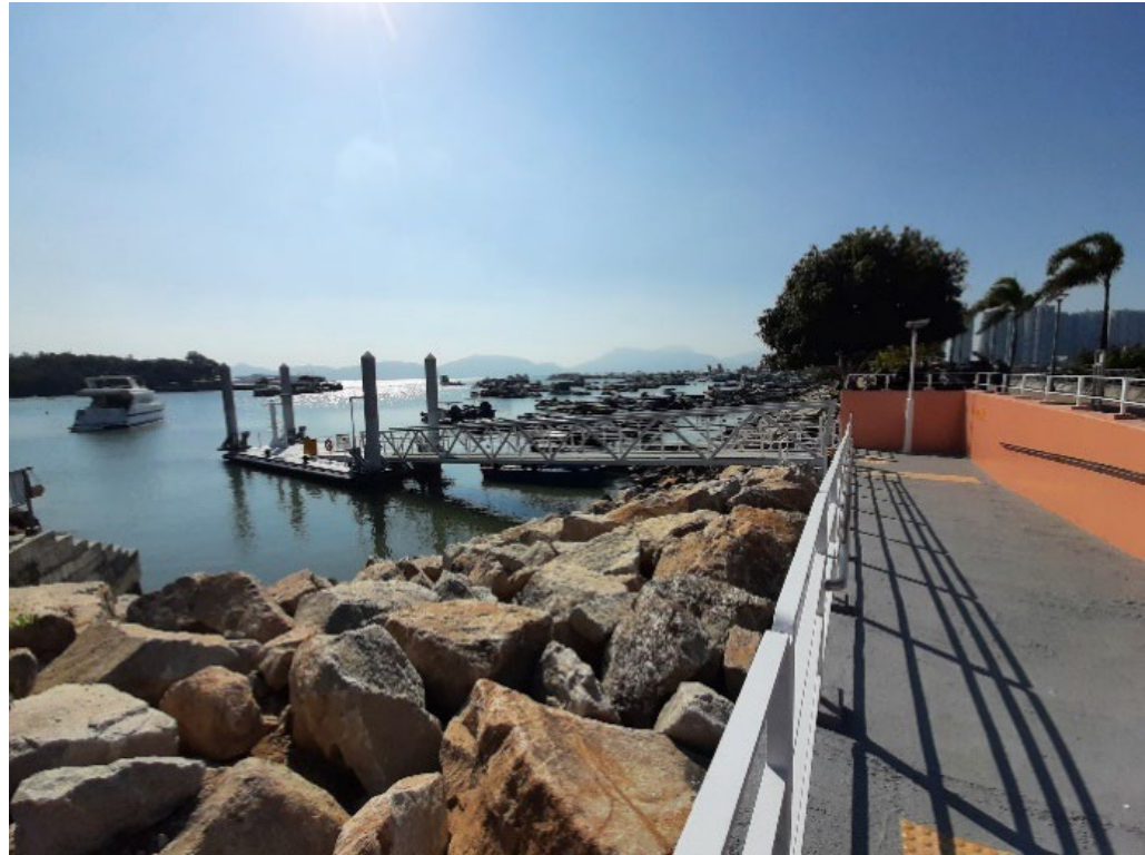
Example: Floating pontoon at Tuen Mun Area 27
