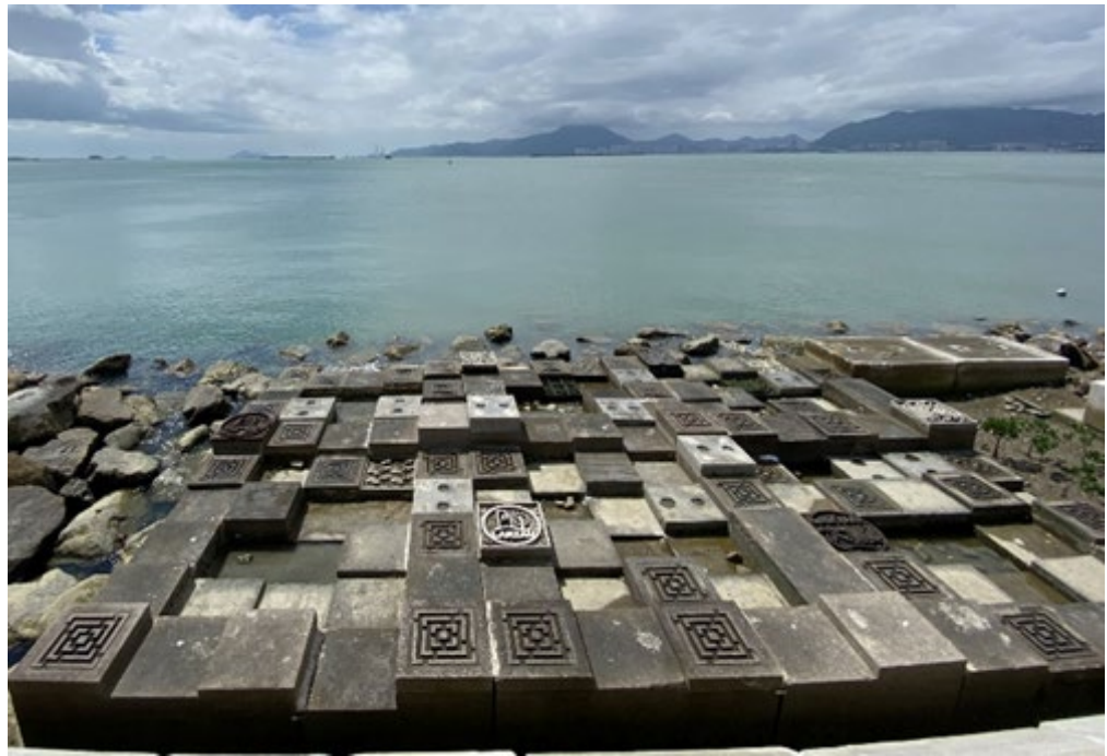
Example: Eco-shoreline at Tung Chung (bio-blocks)
